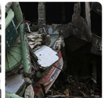
For poor condition
